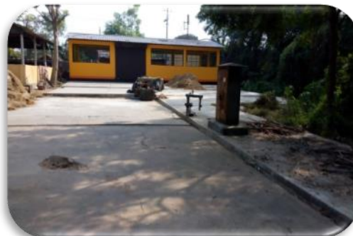
Covered Threshing Floor
