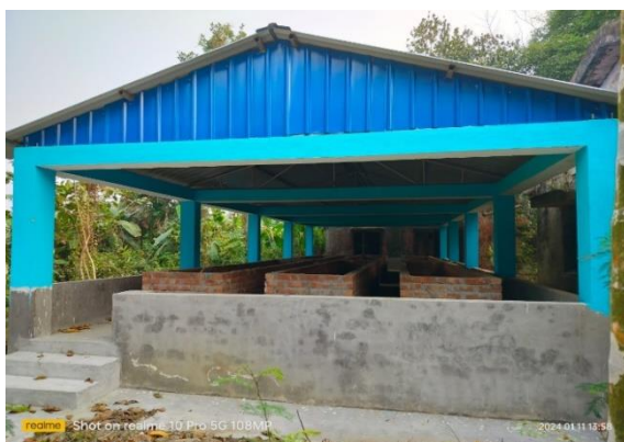
Compost sheds under RKVY
