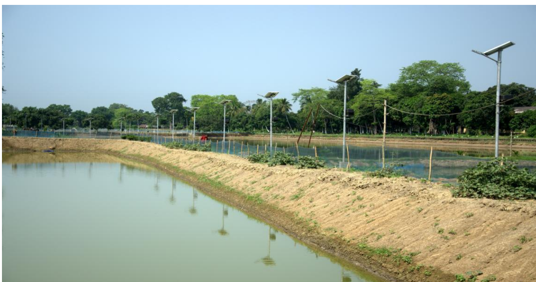
Solar light at Mondouri Farm
