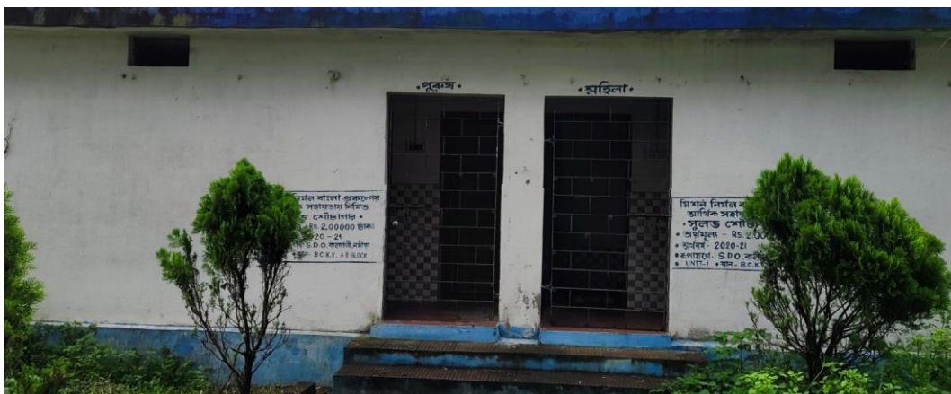
Sanitary complex under Nirmal Bangla Project
