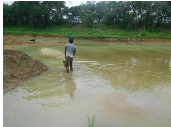
Renovation of farm pond
