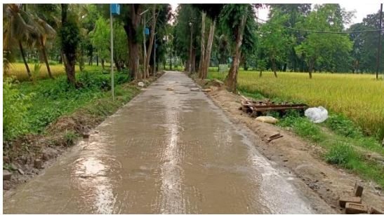
Construction of farm-Road under RKVY project
