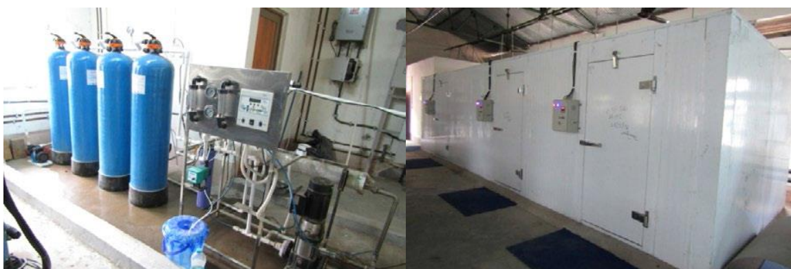
RO plant to supply of soft water to SAVARS cooling chambers made by PUF panels for storage of fruit and vegetable
